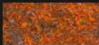
Without corrosion protection treatment
